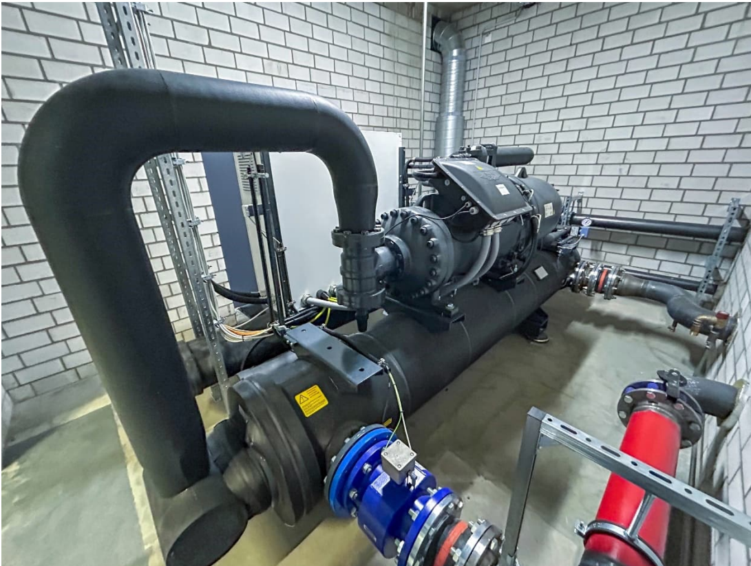
Central unit: the new heat pump. With a thermal output of 622 kW, it is 75 times more powerful than a standard heat pump in a detached house.
